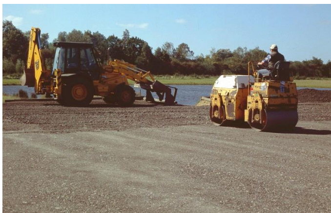
One of the last things to be done before the official opening day was to re-surface the car park using road plannings. Dave Mainwaring driving the roller. 7 September 2004
