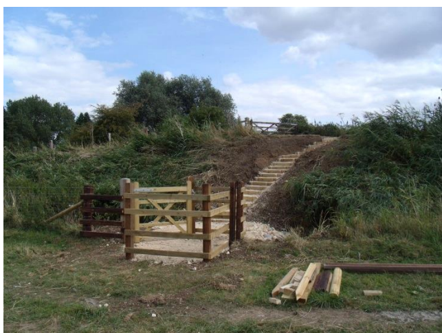
A separate work party, but at around the same time, was installing a new 14' gate on to the river bank. Digging the post holes was difficult – lots of stone in the gateway 14 August 2013
