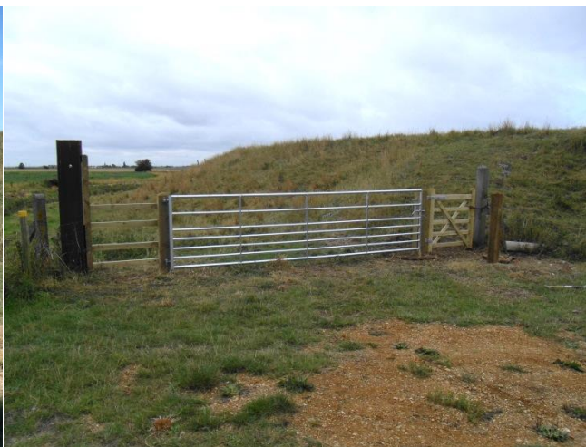
A separate work party, but at around the same time, was installing a new 14' gate on to the river bank. Digging the post holes was difficult – lots of stone in the gateway 14 August 2013
