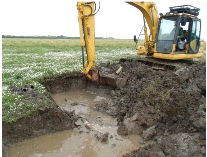
Interceptor ditch working for the first time, with the improved bund, and we found/blocked more old field drains. 26 August 2013
