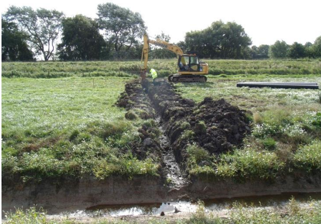
Most of the trench could be dug by machine under close supervision; the bit over the pipe had to be done by hand. 16 September 2013
