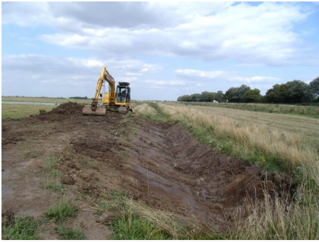
Interceptor ditch working for the first time, with the improved bund, and we found/blocked more old field drains. 26 August 2013
