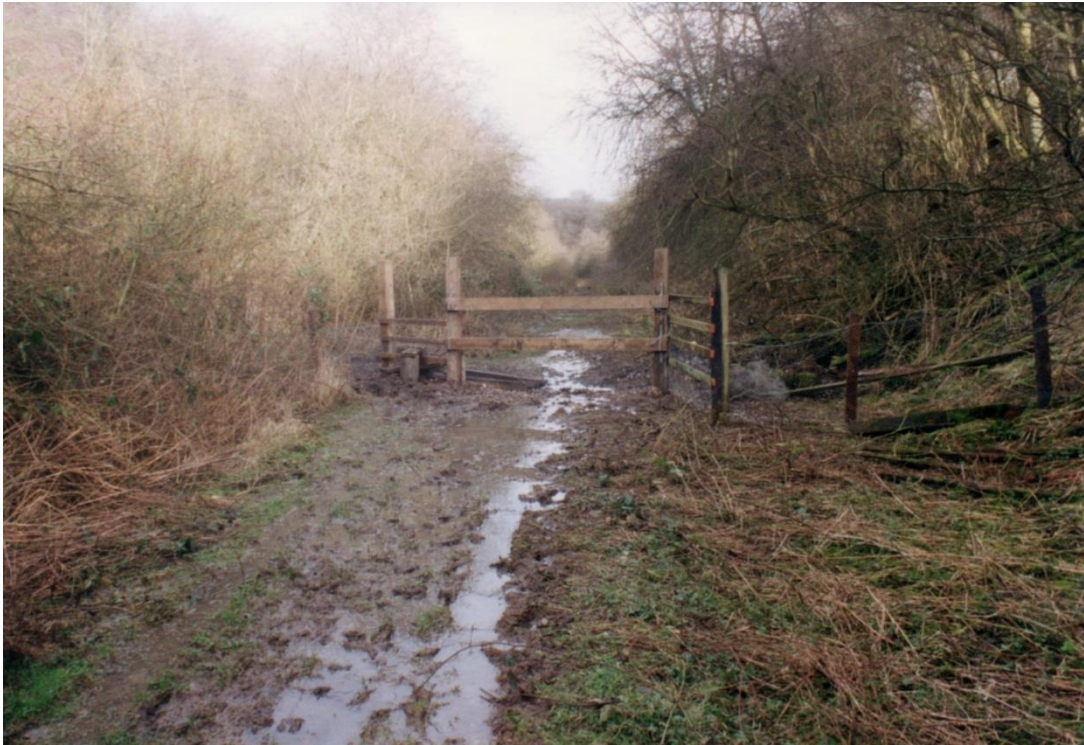
The very muddy conditions were caused by an overflowing ditch on the north side of the cutting, creating a flowing stream along it.
