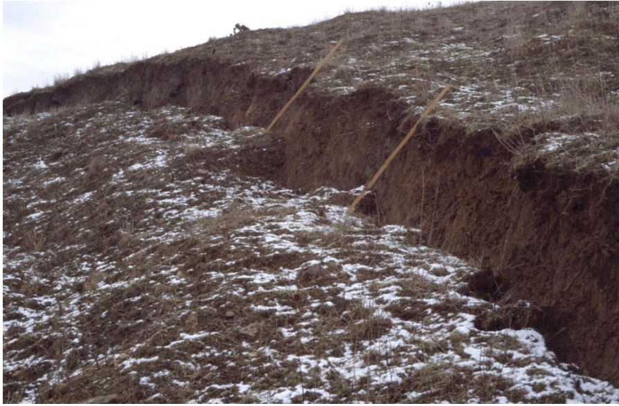
After a particularly wet winter the taller of the two spoil heaps developed a land slip. Photo includes two metre long sticks to indicate scale. 6 February 2003
