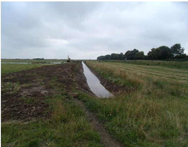
Interceptor ditch working for the first time, with the improved bund, and we found/blocked more old field drains. 26 August 2013
